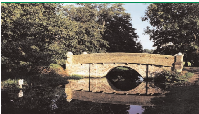
Tewin Meadows bridge (HCC Landscape Unit)
