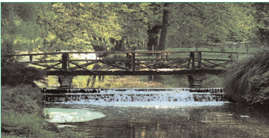
Footbridge over Tewin Water (P. Cullens)
