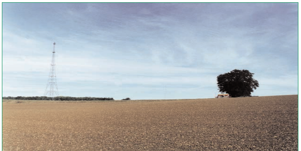
Transmitting station near Hamels Park (HCC Landscape Unit)
